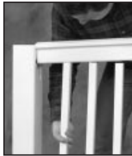
Pull up on the first few balusters and insert them into the top rail holes.
