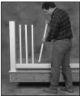
Insert balusters into bottom rail.
