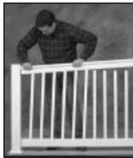
Push down on top rail and position next to the opening. The rail may not fully enter into the opening until you have inserted more balusters.
