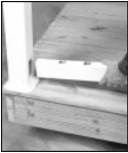
Insert bottom rail into post.
