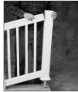
Lift the partially assembled section and insert top rail into opening. Push section down to deck.
